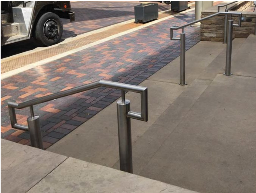
ESCUTCHEON PLATES 100A (STAINLESS STEEL-ASTM A316L)
